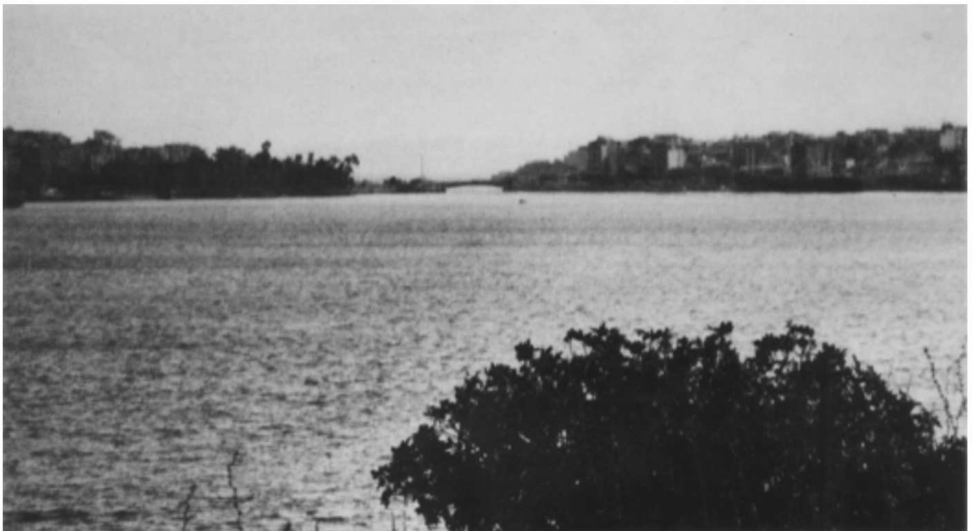
Figure 2. Chalcis bridge from the south.
